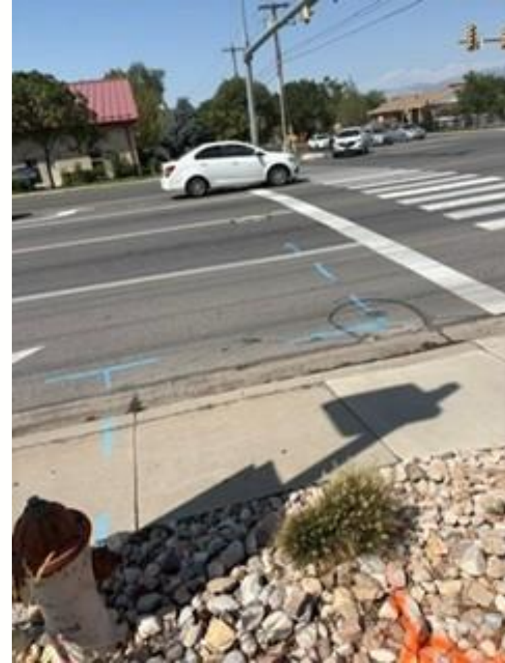
Waterline blue stakes
