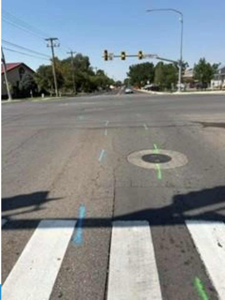
Water and sewer main blue stakes
