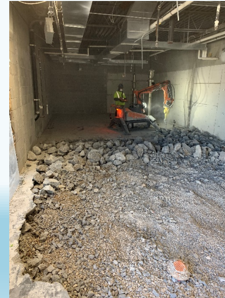
Compacted base material for footings and interior concrete subfloor demolition
