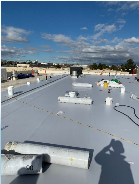
Roofing Membrane Installation
