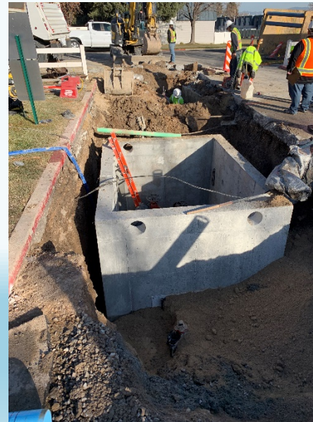
Meter Vault Installation at Wildwood Cove
