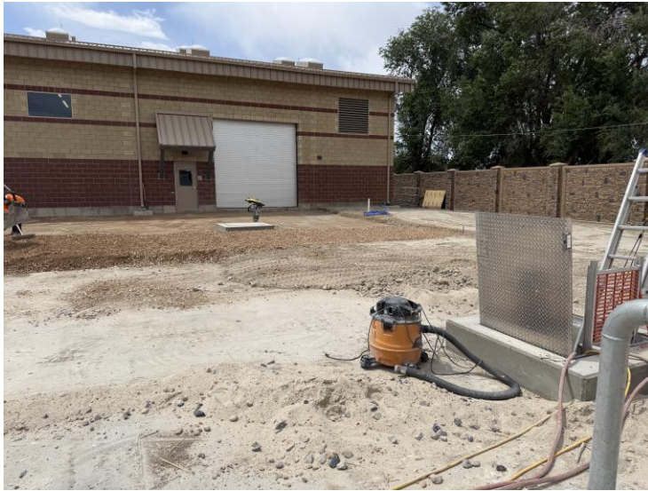
Anderson WTP Backwash Basin backfilled and covered for driveway and landscaping install
