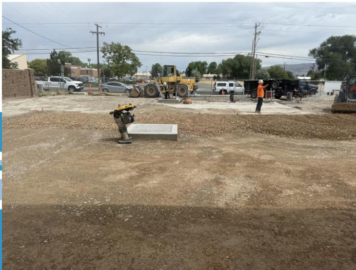
Anderson WTP Backwash Basin backfilled and covered for driveway and landscaping install
