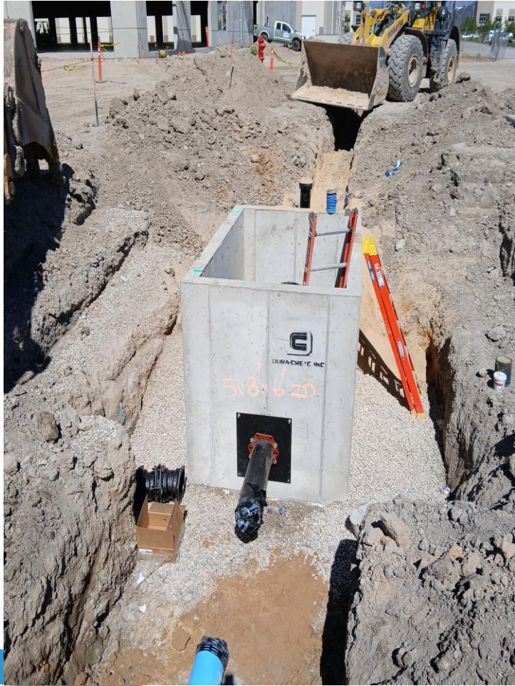
DCDA vault install
