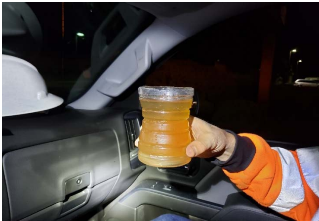
Fig. 1: Water sample taken during flushing
