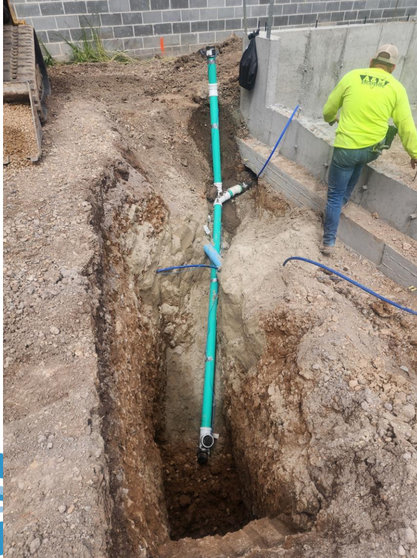
4" sewer lateral inspection for new home construction
