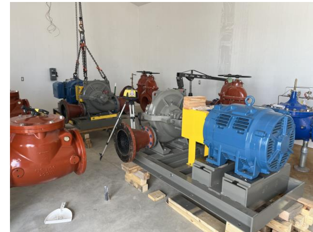
Booster pump installation.
