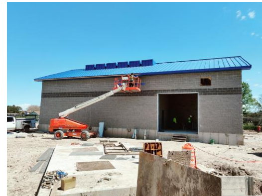
Worker applying finishing touches to the roof
