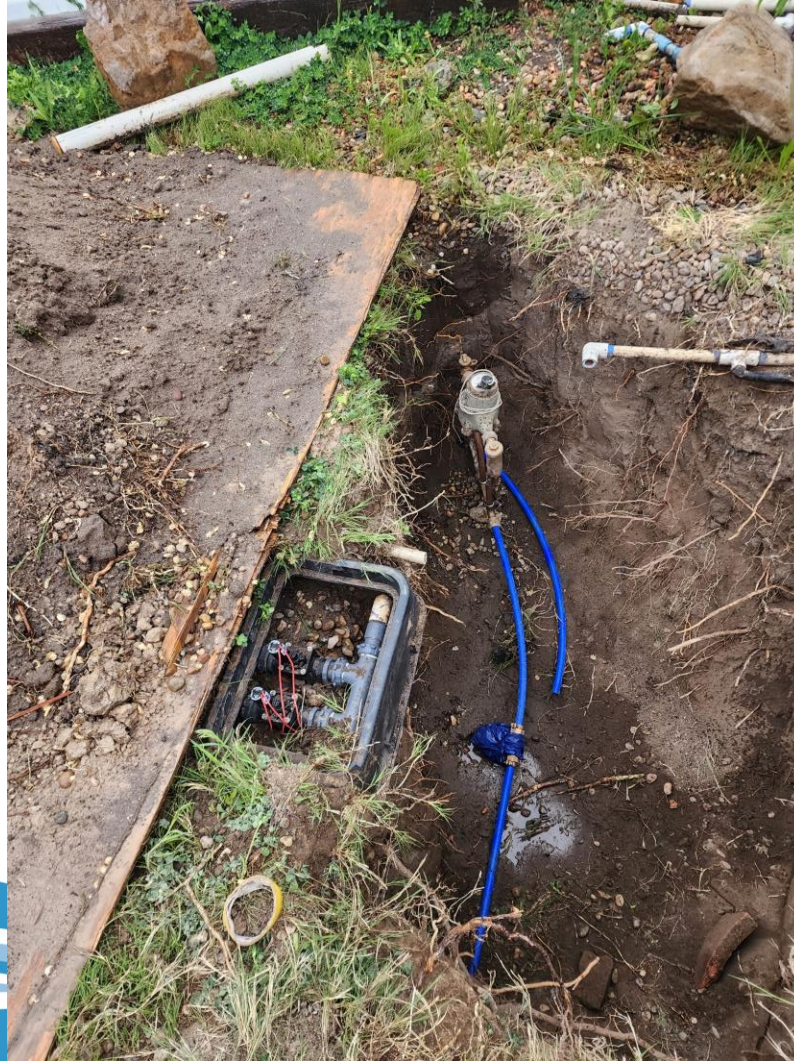
New water lateral installation
