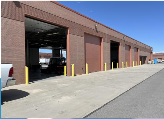
Newly installed garage doors in operation
