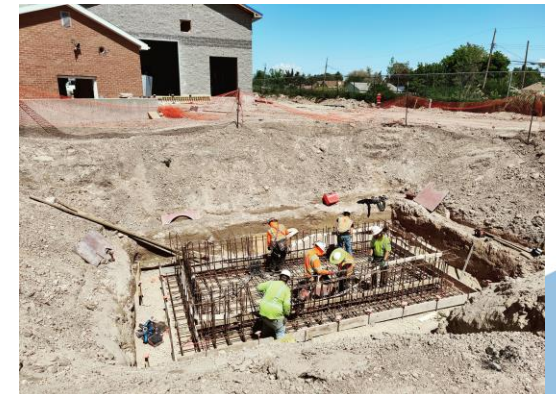
Installing rebar for surge tank vault
