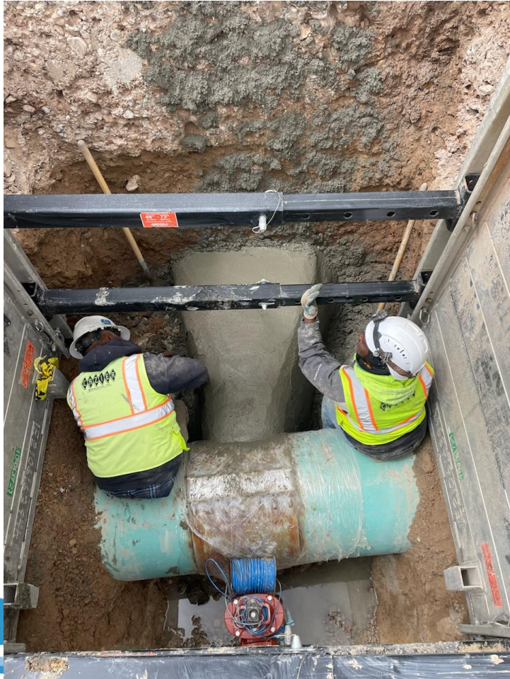
4" tap on 24" water main with thrust block
