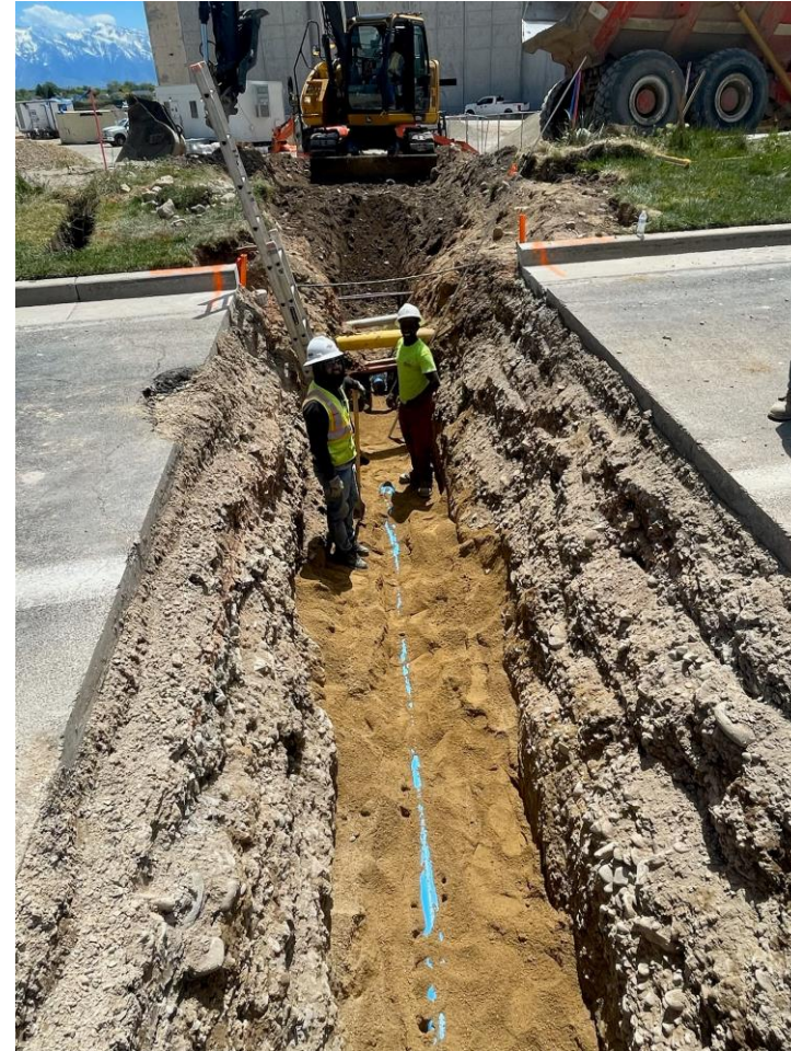
4" water lateral trench
