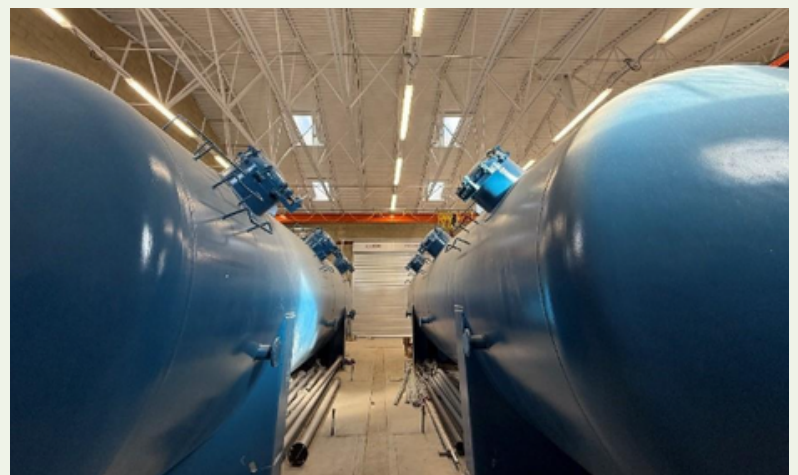
Photo: Filter vessels in new groundwater treatment plant
