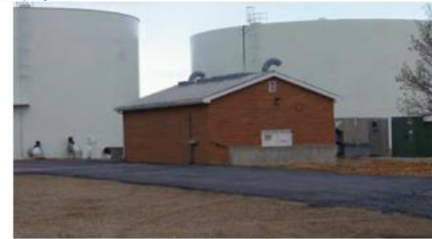
Kent Pump Station
