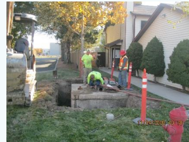
Removing the existing Stone Creek Meter Vault
