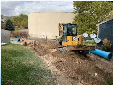
Pipe installation near Mulberry Apartments
