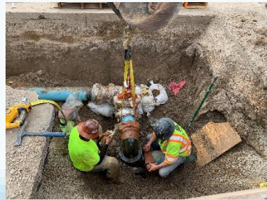
Applying wax tape on fittings
