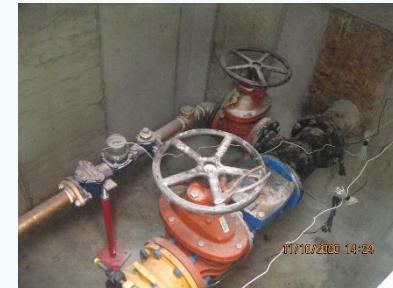
Inside the new Stone Creek Meter Vault
