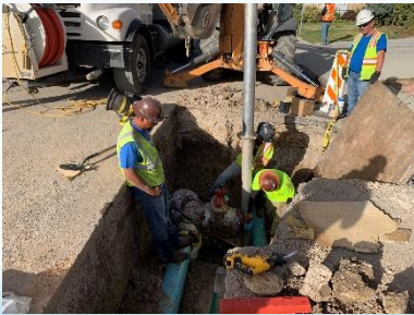
Draining existing waterline for tie-in on Bird Song Road
