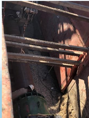
Installing steel casing under canal using jack and bore method
