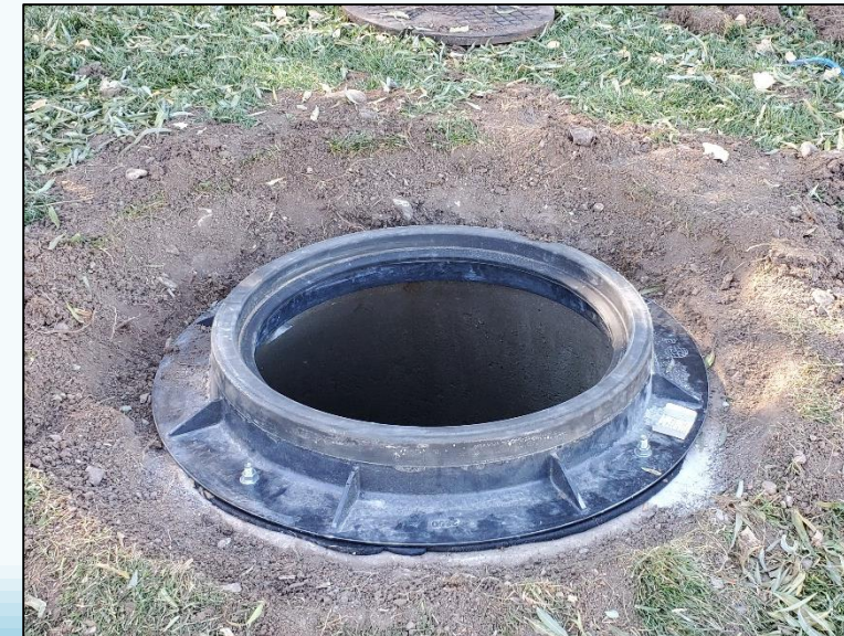
Depicts manhole frame changed out to an anchored down composite style.
