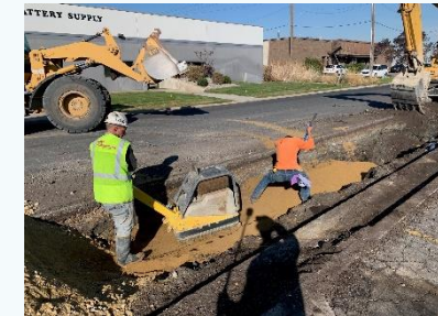
Compacting new 8" pipeline
