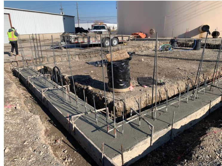
Booster pump station footings.
