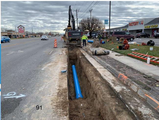
Waterline installation along the west side of Redwood Road near 3500 South.
