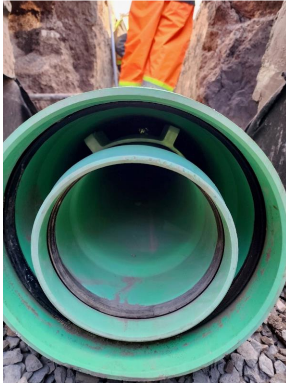
10" sewer main with spacers inside 15" casing
