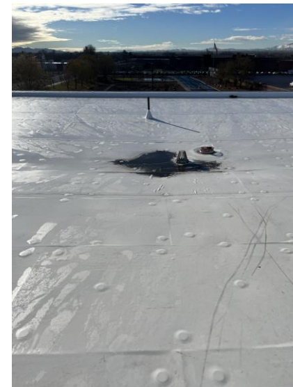
Newly installed membrane
