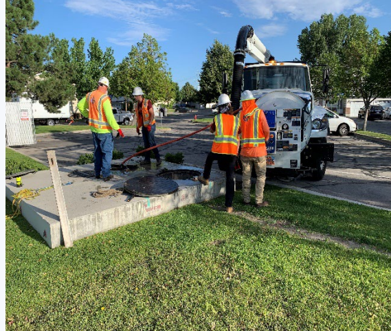
Crew's cleaning the CVWRF meter pit from the diversion box.
