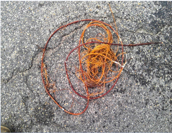
Roots removed from main line
