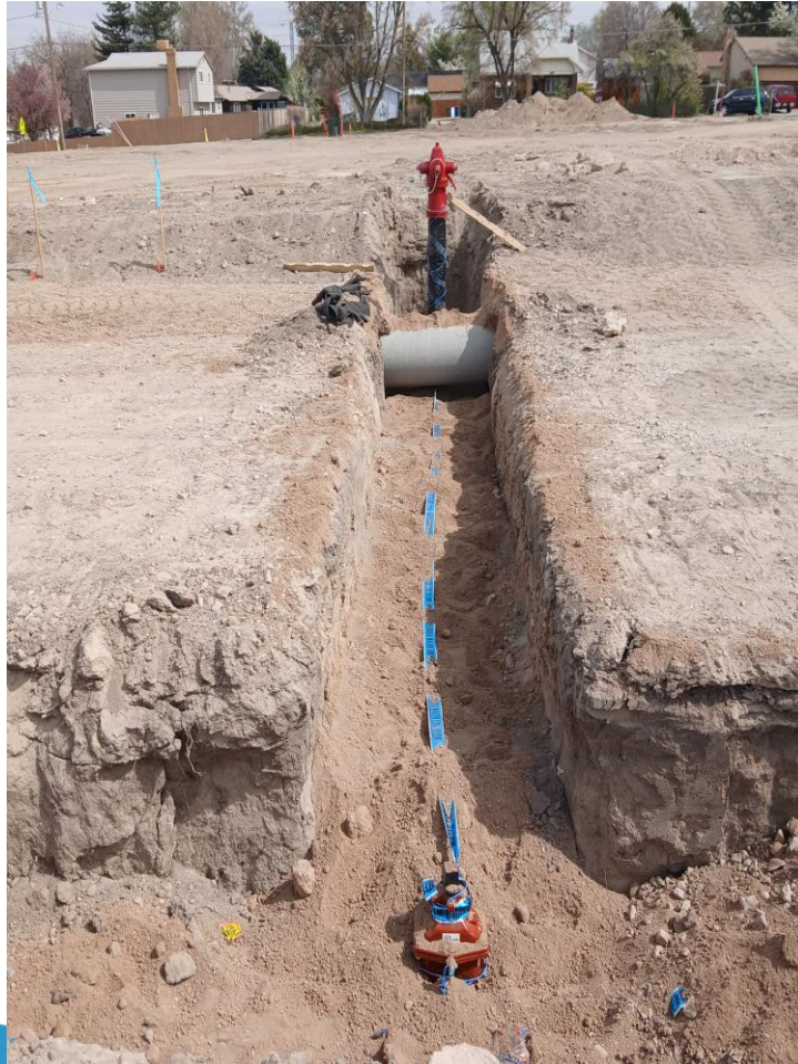
Fire hydrant trench
