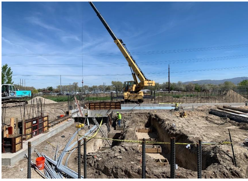
Interior Footings and Electrical Conduit
