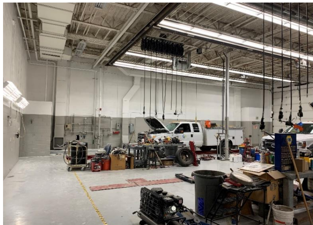
Building Remodel - New Paint in Shop Area
