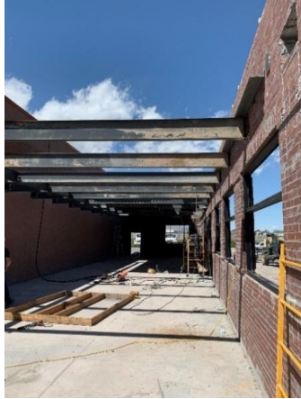
Building Addition - Beams and Decking
