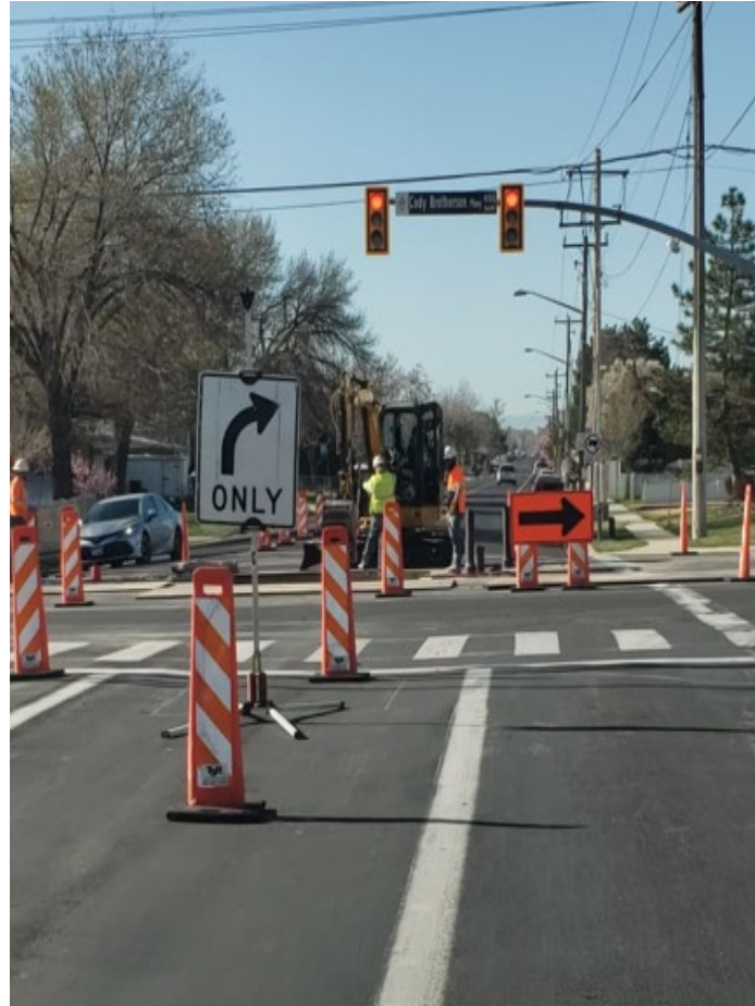
Figure 2: View of job site looking South on 2200 West 4100 South.
