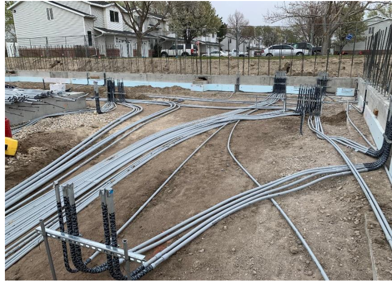
Interior Footings and Electrical Conduit
