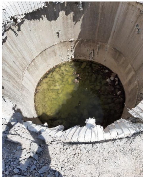
Wet Well Backfill Preparation
