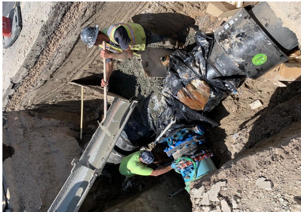
Thrust block behind 28-inch HDPE Tee
