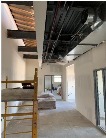
Building Addition - Drywall and temporary skylight cover
