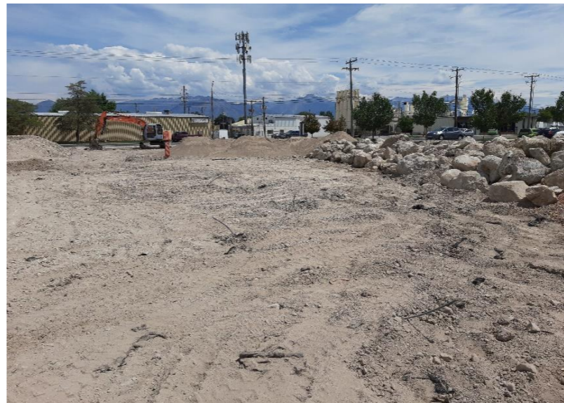
Grading along the south side of property
