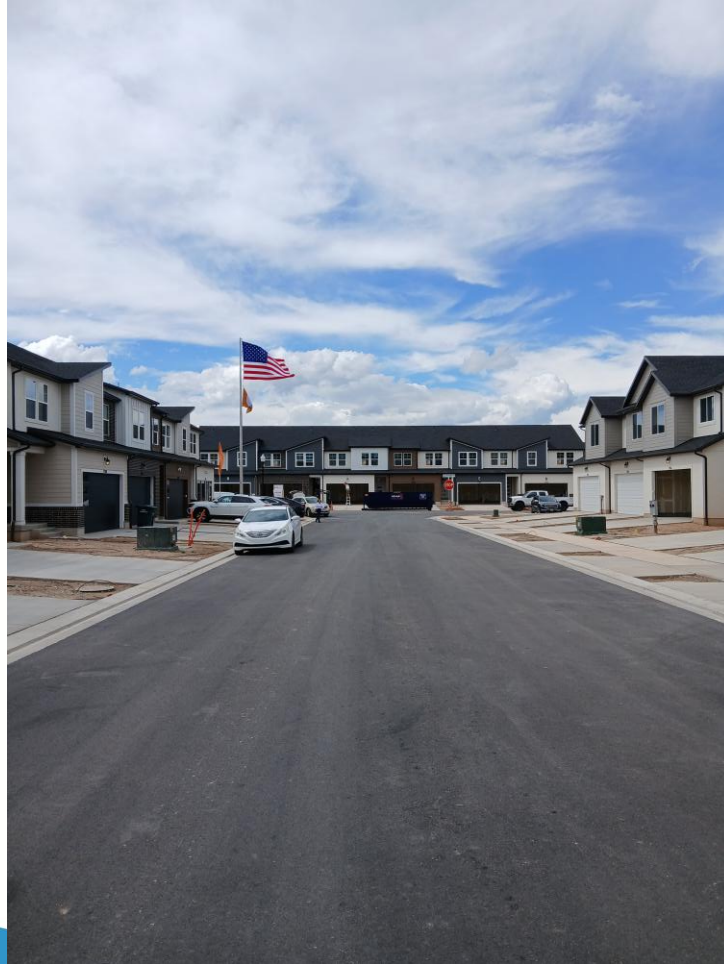
Phase 1 development progress
