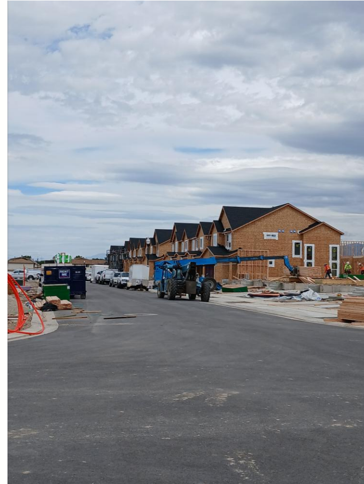
Phase 3 development progress
