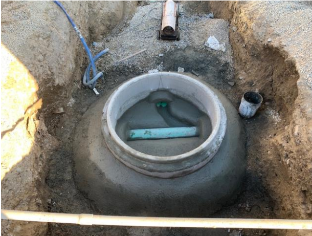
Cast-in-place sewer manhole for 8" sewer
