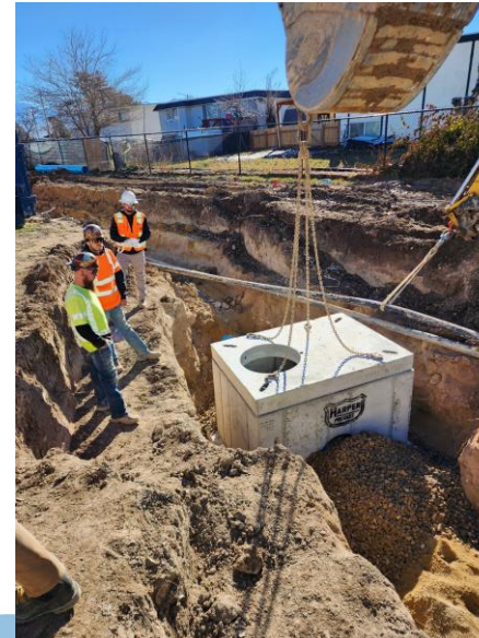
Placing lid on air/vacuum release assembly vault
