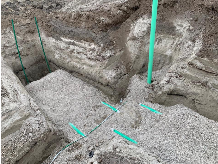
4" sewer laterals with gravel bedding and underground warning tape
