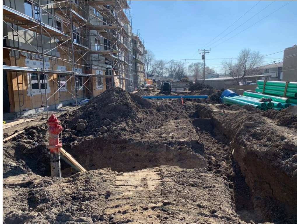
Newly installed fire hydrant
