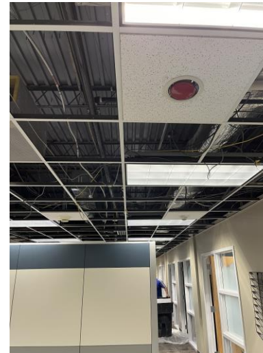
Ceiling Tile Removal
