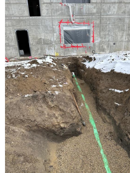
Sewer pipe on west side of building
