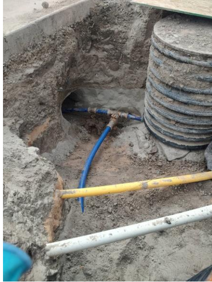
Temporary 2" water lateral installed before existing meter
