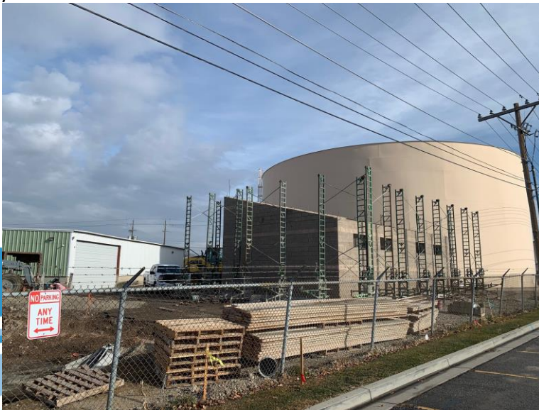
Booster pump station CMU wall installation
