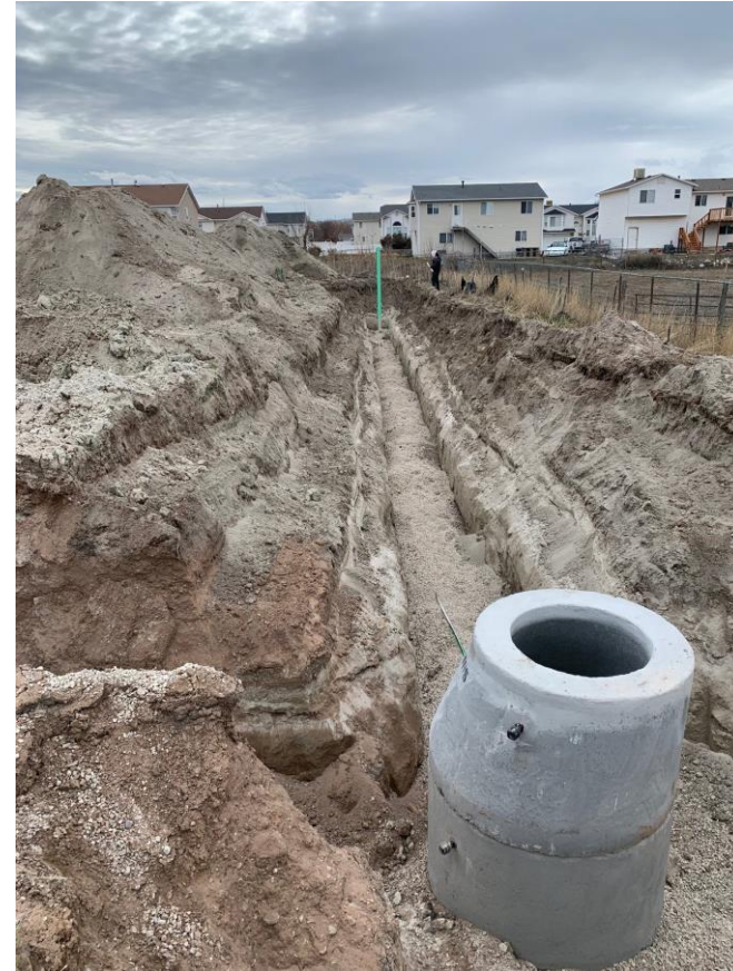
View of sewer trench and manhole
