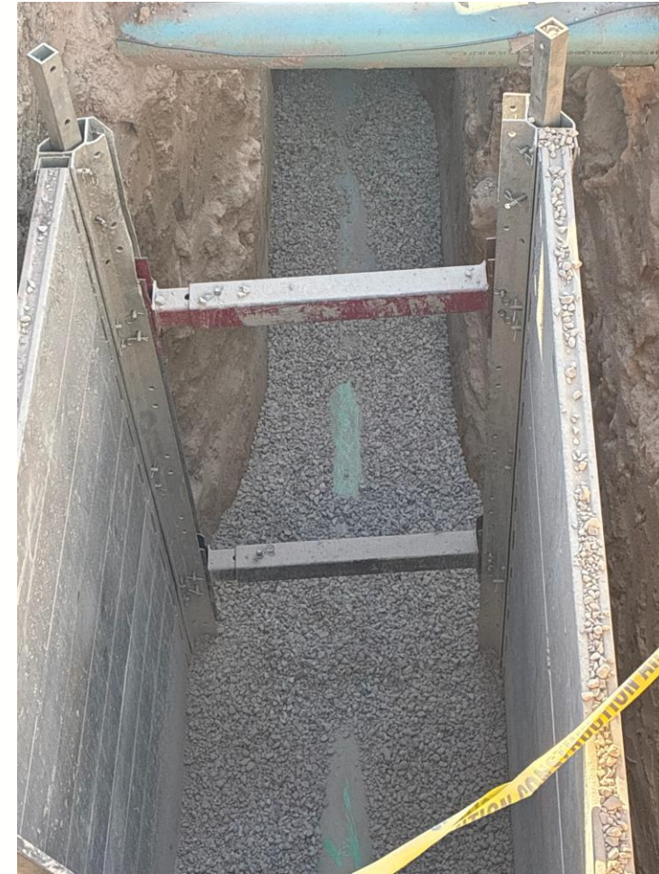
8" sewer main bedded in gravel
