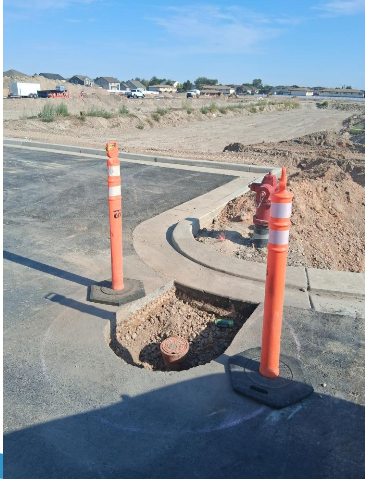
Fire hydrant valve collar prep
