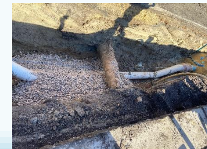
8" prefabricated loop installed under existing sewer main at 2159 W. 2200 S.
