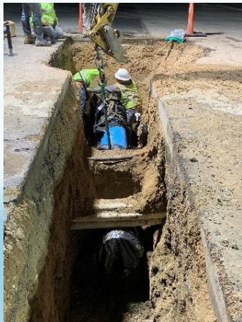
4700 South tie-in. Work done at night.
