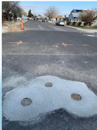
Raised valve boxes at a 'tee'
