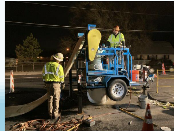
Preparing liner for insertion into existing sewer line.
