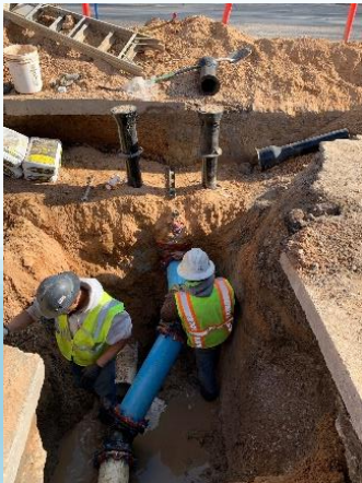
8" Tie-in at August Field Drive
