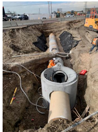
Installing West Valley City's 36-inch storm drain
