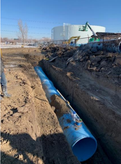
36-inch PVC Installation
