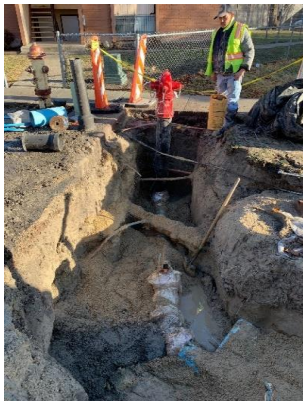
Fire Hydrant Installation
