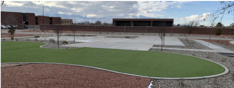
Finished concrete pad for demonstration garden area
